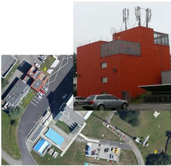
FIGURE 2.10 – Station de base Orange
