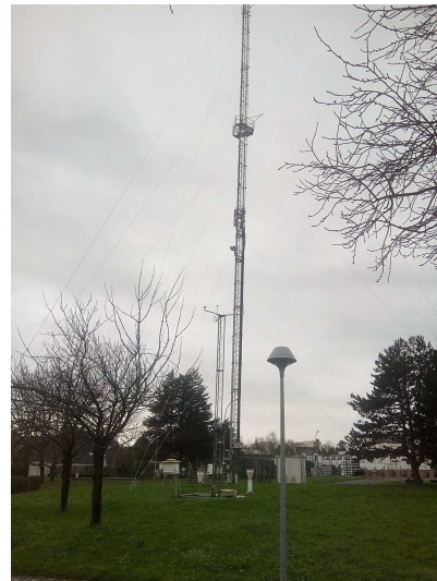
FIGURE 2.11 – Station de base SFR
